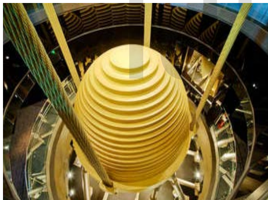
Fig. 2 Tuned mass damper
